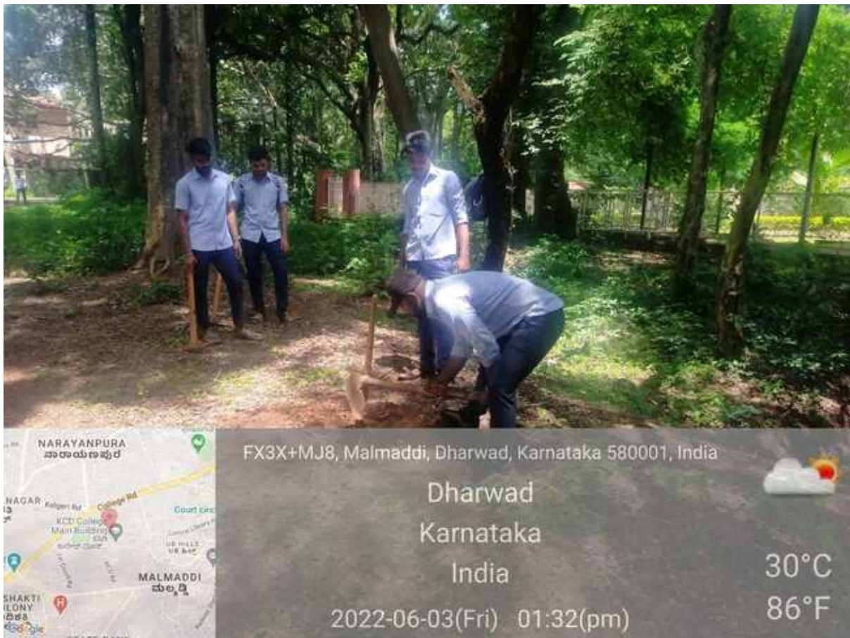
Digging Fits And Campus Cleaning.
